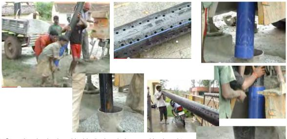
4. Once the pipe is placed inside the borehole, gravel is placed to fill the space around the hole. Stormwater can now be oriented to it.
