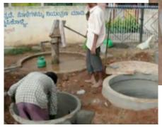
3. The 2 rings on top of the concrete slap are filled with 20 centimeters filtering medias: Here (from the top of the slab to the surface):
