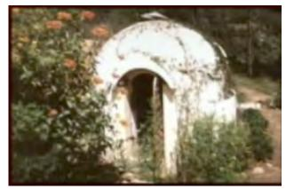
This structure protects a well fed by rainwater harvested from several rooftops to a quantity of 270 m<sup>3</sup>. The Barefoot College built rainwater fed wells in 500 schools and estimated the annual collection of 300,000 Million liters. They also built 100-feet diameter open wells allowing to collects 1 Million liters rainwater.
