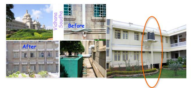
Figure 6. Example of retrofitting buildings for rainwater collection
