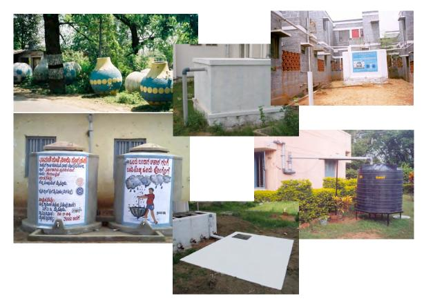
Figure 4. Options of rainwater storage containers
