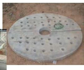
on top and then 2 more rings are placed on top of the perforated slab to act as a filter. The photo below shows the man standing on top of the concrete slap and installing the 2 additional rings above the slab
